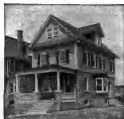
A No. 1-19-S IDEAL Boiler and 184 ft. of 38-in. AMERICAN Radiators, costing the owner $106, were used to heat this cottage. At this price the goods can be bought of any reputable, competent Fitter. This did not include cost of labor, pipe, valves, freight, etc., which are extra, and vary according to climatic and other conditions.
