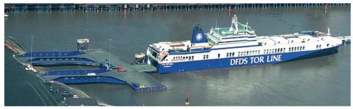
The MacGregor linkspan can accomodate up to three ships side-by-side with various stern ramp configurations, all loading and discharging simultaneously. The pontoon is connected to the shore terminal by two three-lane bridges.
